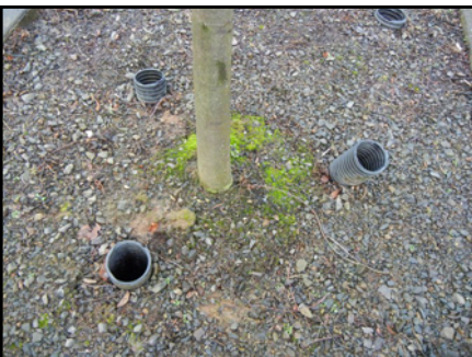
Fig 2: Plastic tubes installed at planting time for the purpose of "aerating the root zone." And yes, the tree is planted too deep.
